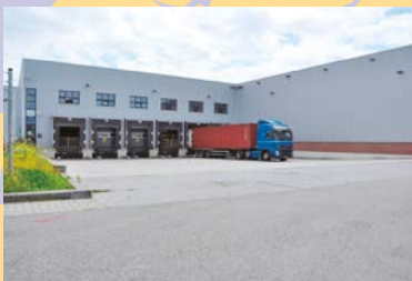
Netherlands (European Distribution Centre: EDC)
